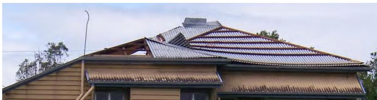
FIGURE 2. PART OF THE ROOF CLADDING WITH BATTENS STILL ATTACHED FLIPPED ON TO LEEWARD SIDE
