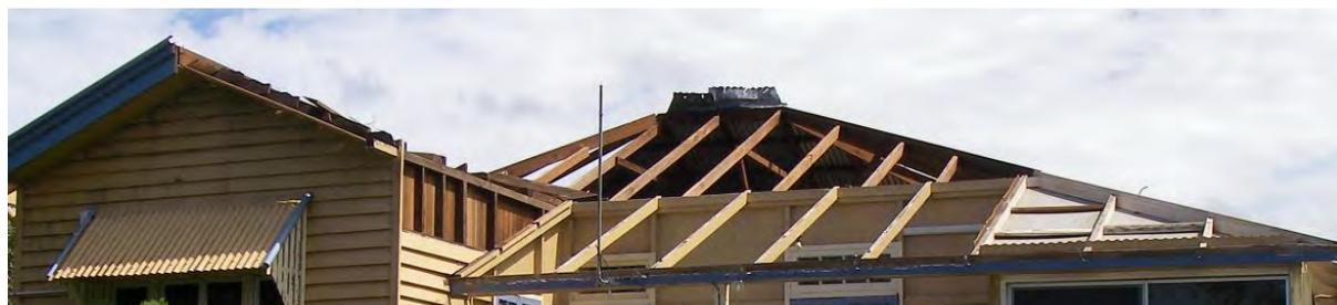
FIGURE 1. REMOVAL OF ROOF CLADDING AND BATTENS FROM WINDWARD FACE
