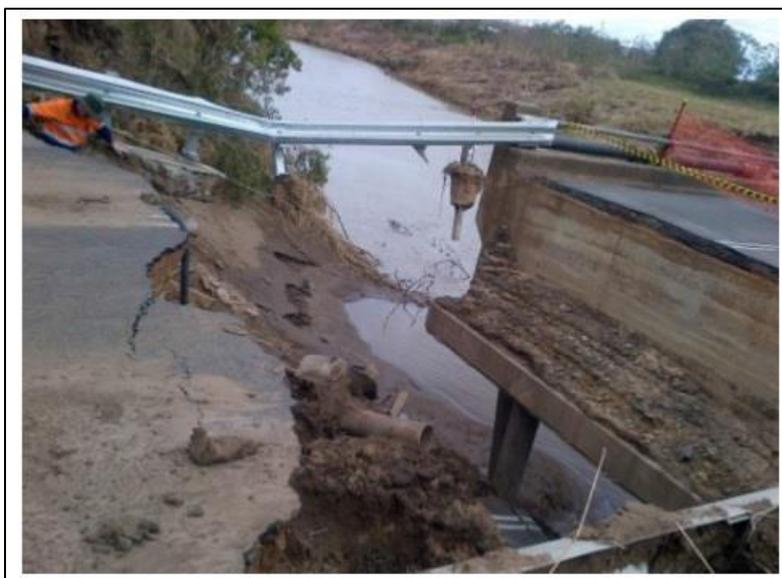
Figure 2.29: Abutment washed away on Gatton-Esk Road bridge (Ezeajugh, 2014)
