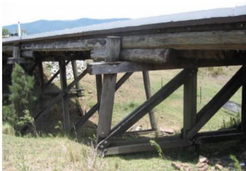
Figure 2.19: New Country Creek bridge near Kilcoy, timber girder bridge (Eyre et al., 2012)
