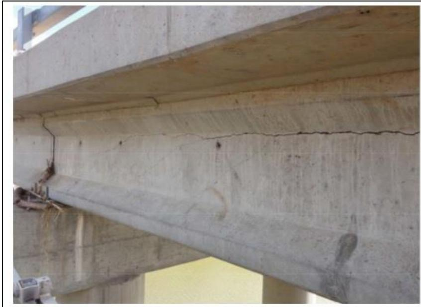
Figure 2.28: Damage to Kapernicks Bridge (Cracking in girder) (Murray and Kemp, 2011)
