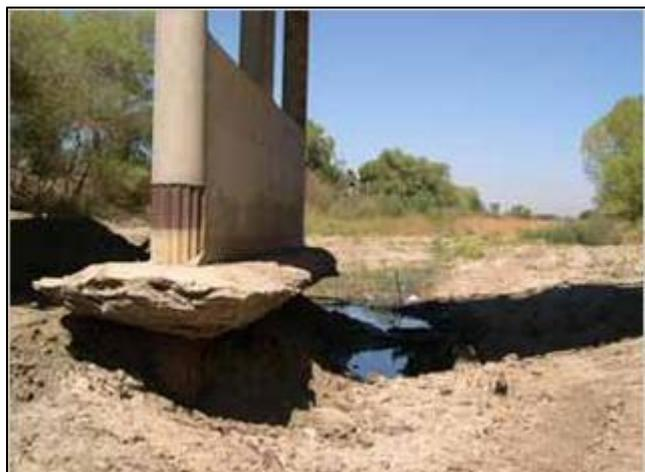
Figure 2.24: Scouring around a bridge foundation (Lin et al., 2010)
