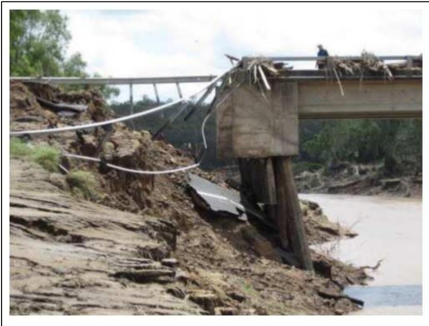
Figure 2.27: Damage to Kapernicks Bridge (Approach washed away) (Murray and Kemp, 2011)
