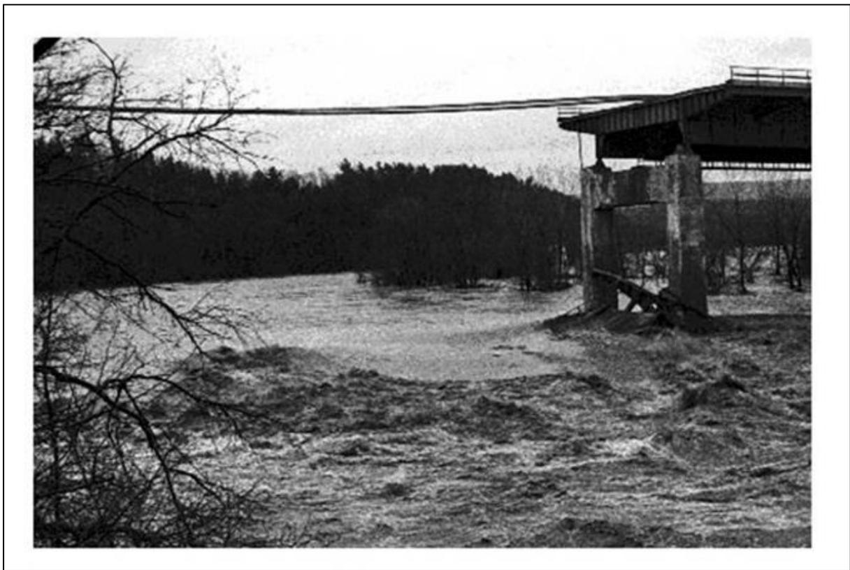
Figure 2.21: Collapse of the Schoharie Creek Bridge due to flood in 1987 (reprinted from USGS 2012)
