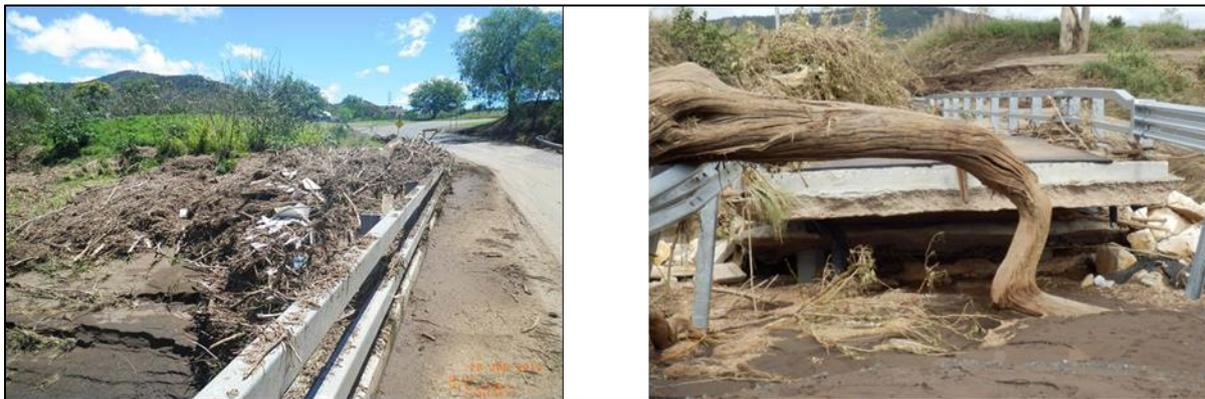
Figure 1.1: Damaged Bridges in Lockyer Valley Region in Queensland (The Lockyer Creek Flood of January 2011)
