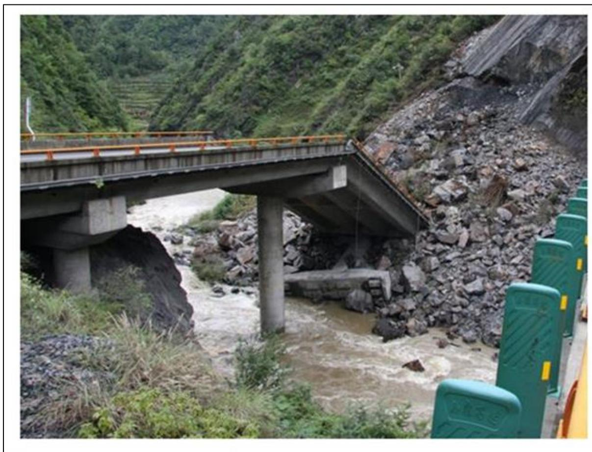
Figure 2.22: Collapse of a bridge due to landslide (image courtesy of (Zhong et al., 2013))
