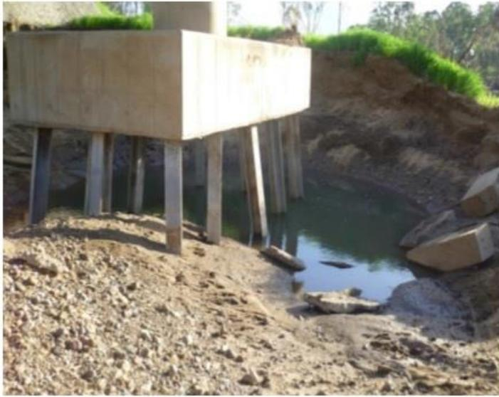
Figure 2.30: Scour around pier and exposed piles on Geoff Fisher Bridge (Ezeajugh, 2014)
