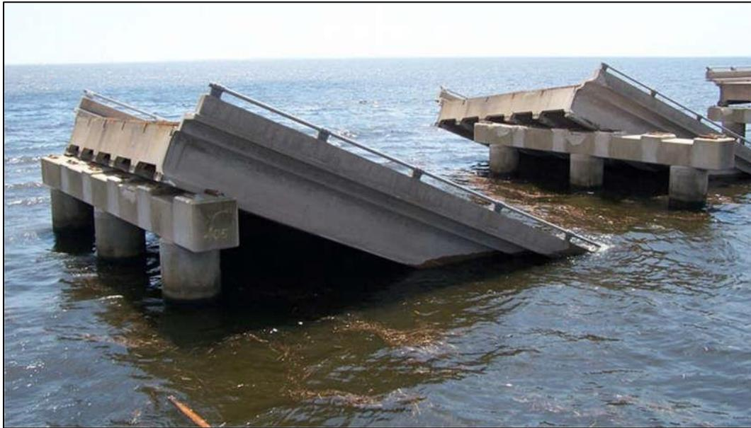
Figure 2.23: Bridge collapsed under Typhoon
