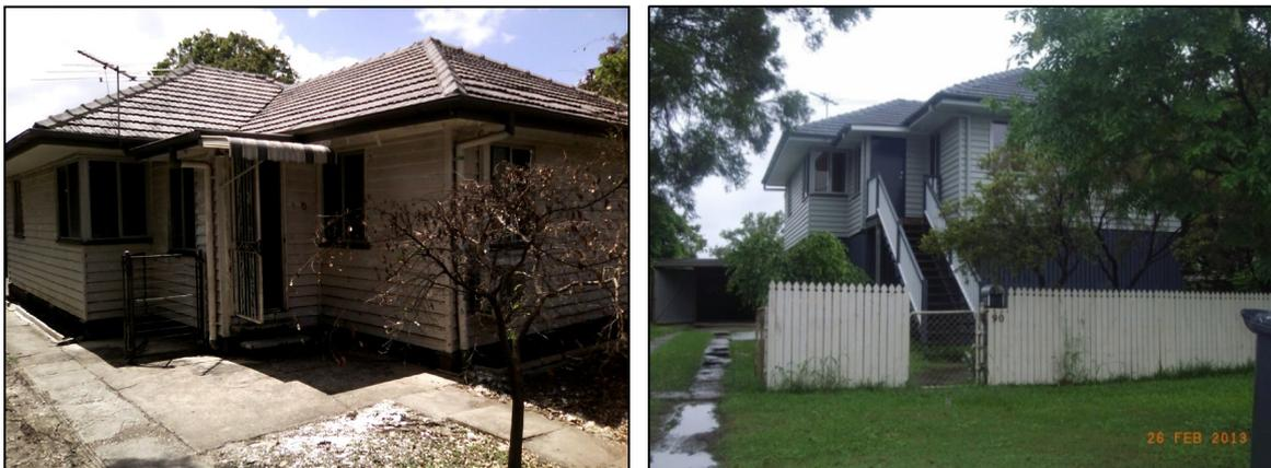
FIGURE 3: AUSTRALIAN EXAMPLE OF MITIGATION THROUGH ELEVATION
