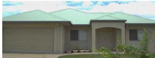
Reinforced masonry block, hip and gable, large truss spans, medium roof pitch, slab on ground
