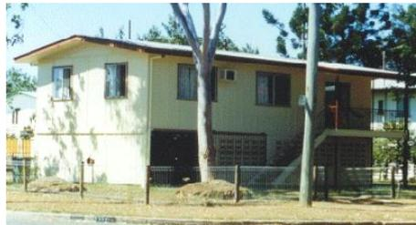
Gable low pitch, vermin proof flooring (studs not mortice and tennon into bearers), panel cladding, on stumps
