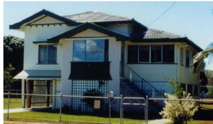
Hip and gable, VJ lining, reduced rafter spans, on stumps (low and high)
