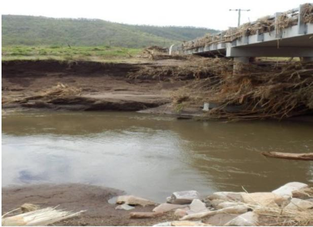
Damage to abutment & headstock
