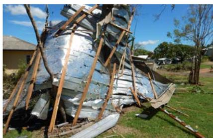
Wind-induced failure of a metal cladding roof at the batten to rafter connection during Cyclone Marcia (2015) in Yeppoon, Australia - there appeared to be no retrofitting of the weaker connections.
