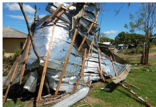
Batten to rafter failure caused by Tropical Cyclone Marcia
