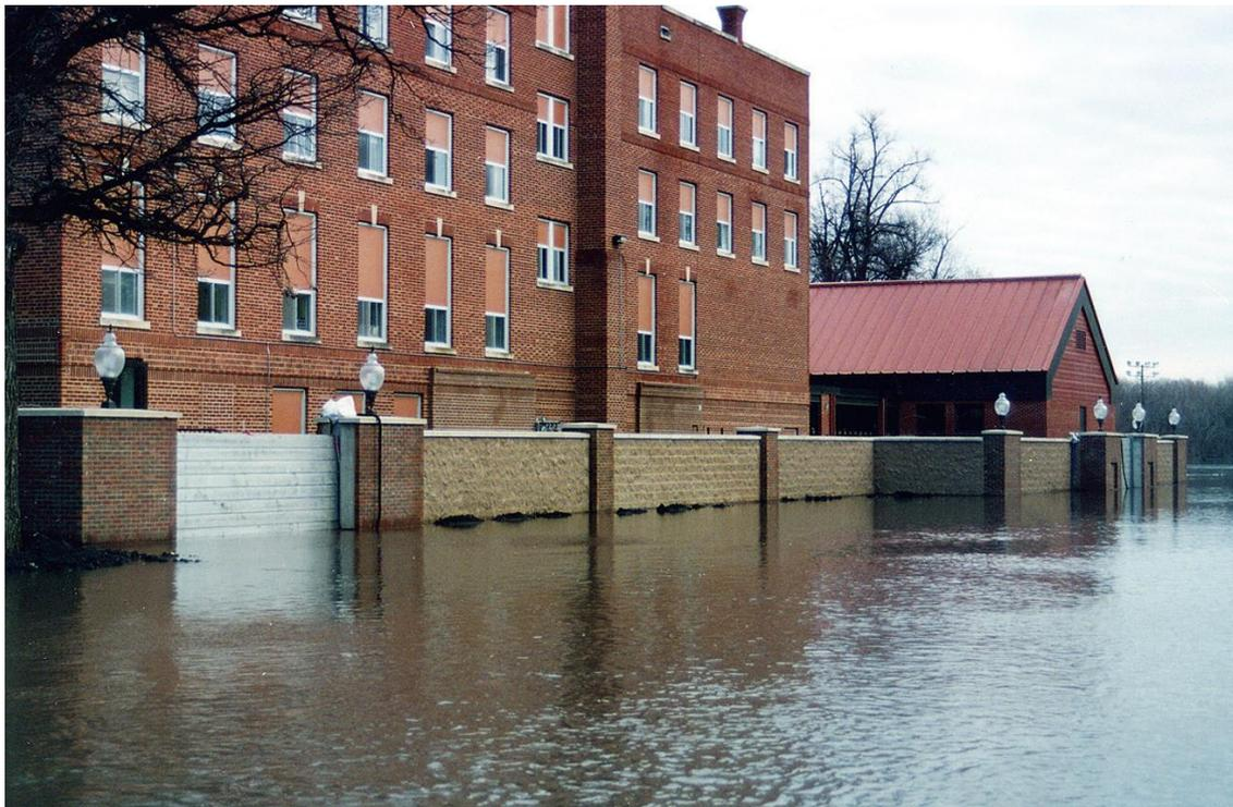
Figure 9. An example of a floodwall (FEMA, 2013)
