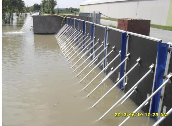
Figure 10. Examples of flood barriers (Bluemont, 2015)
