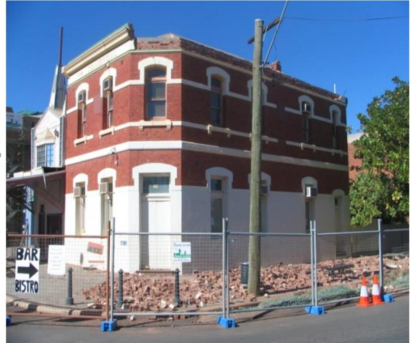
Parapet/awning damage in URM buildings in M5.0 earthquake
